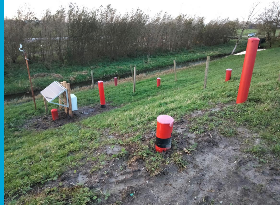
Dyke monitoring at the Duifpolder
